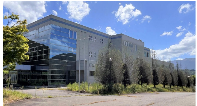
Ueda No. 2 Plant
