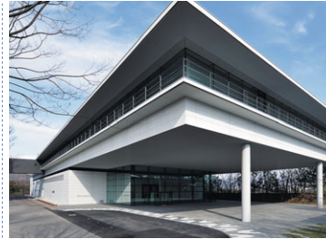
HIOKI Innovation Center, the company's new R&D complex, is completed.
